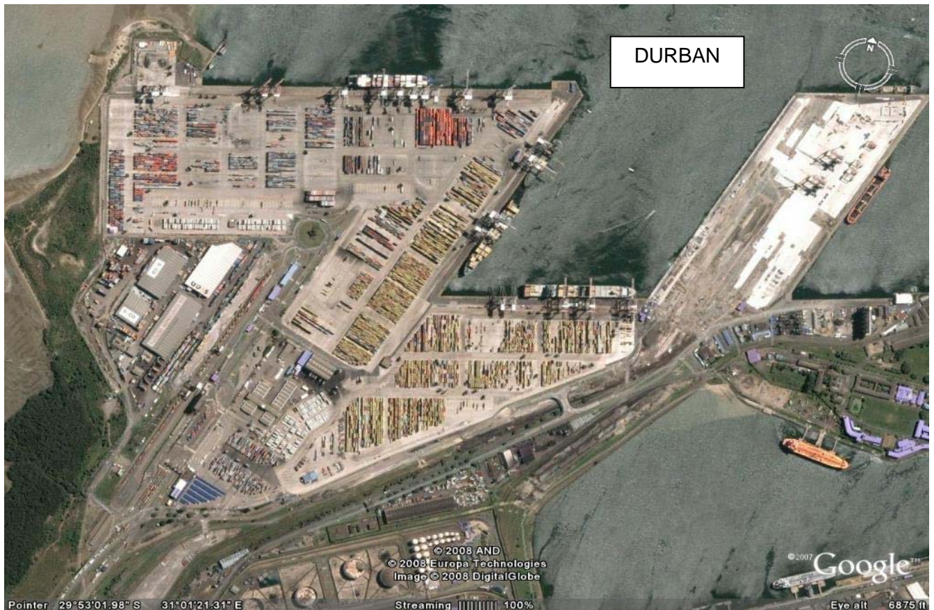
Figure 27: Durban Container Terminal [DCT]
