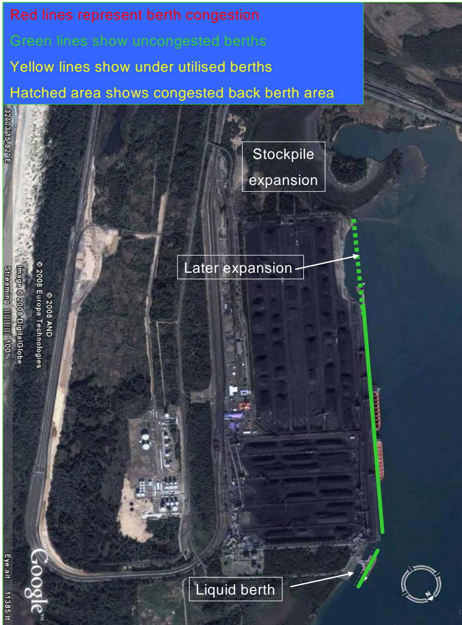
Figure 21: The Coal and Liquid Terminals
